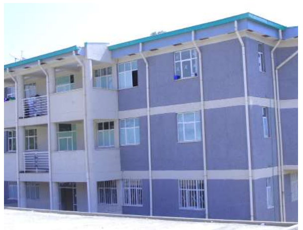
Newly constructed staff's residency.
