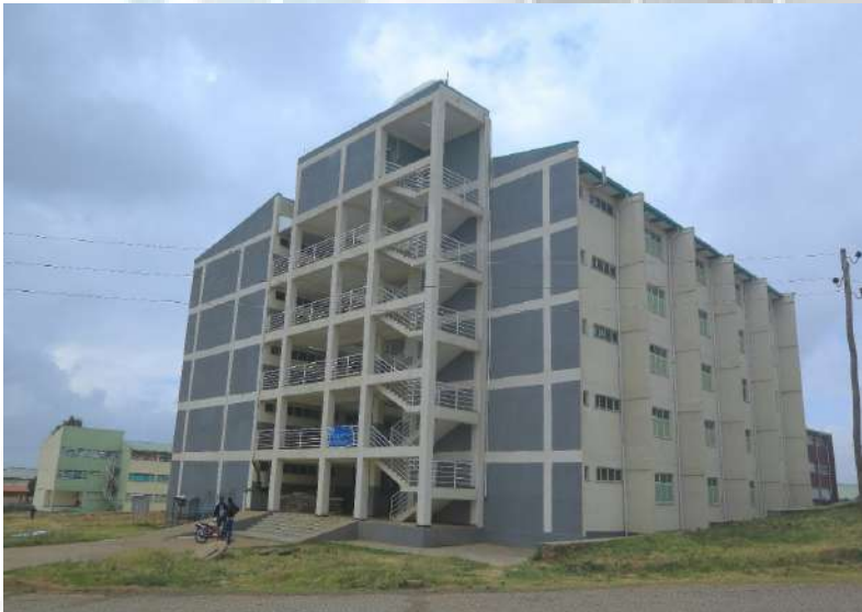
Engineering and Technology Laboratory Building
